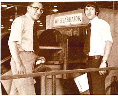
As part of his training schedule, Dave Hanson (right) benefits from the experience of Harold Schulte, Chief Engineer, in starting up the 10-wheel Drum Cleaning Machine at Bayonne Barrel and Drum Co.
